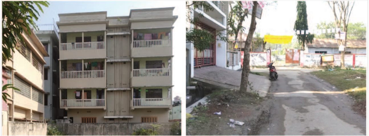
Fig. 2a. Violation of setback regulation, Fig. 2b. Car parking ramp connected to the road
