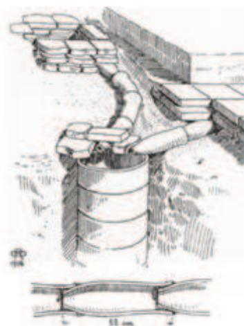
Fig. 3: Waste water disposal into the underground in Assur (Mesopotamia) 2.500 BC (Source: Illi 1987).
