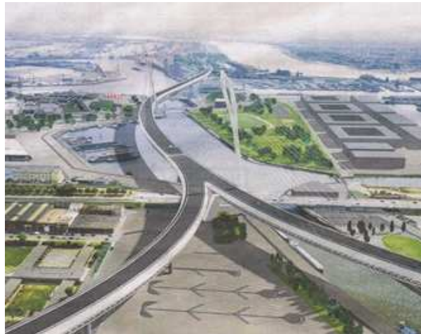
Figure 6: The Lange Wapper' overpass as landmark for the province of Antwerp ( http://www.bavo.biz )
