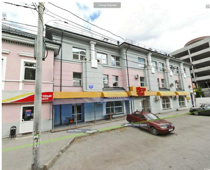
Fig.4 Façade of building, Kirov street.
