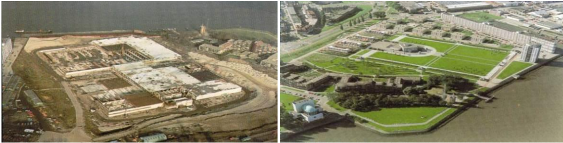
Figure 2a and 2b: Dokhaven redevelopment Rotterdam (NL) before and after completion
