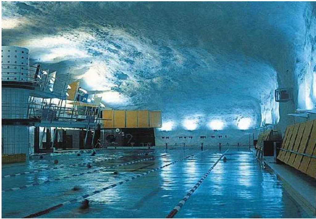
Figure 6: Itäkeskus Swimming Pool, Helsinki (FI)
