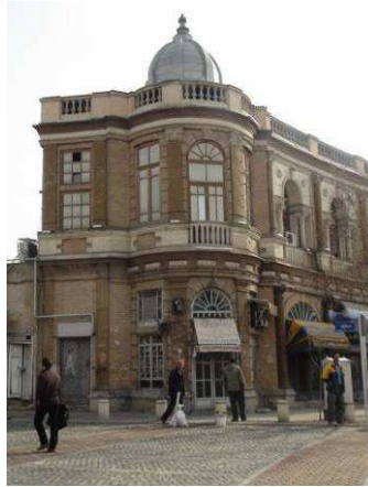
Fig. 11: The north –east façade of Hasan Abad square
