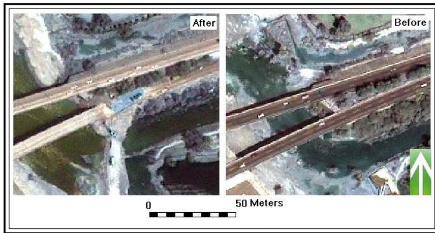
Fig. 6: a damaged part of a bridge on Alqurm area Bridge (left), the bridge before the cyclone (right)
