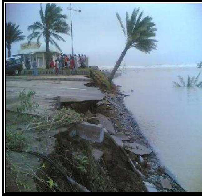
Photo (2) damages on Alqurm beach
