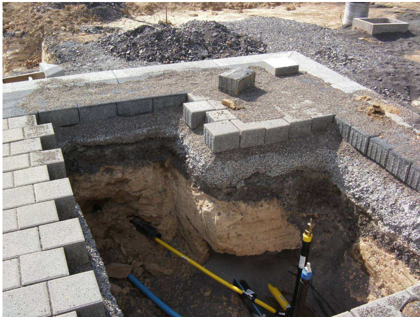
Fig. 3: Infiltration pavement - buildup
